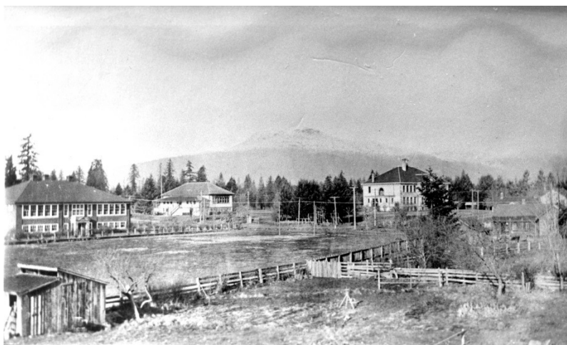
Cairnsmore School, Duncan High School, Duncan Elementary School c. 1932
