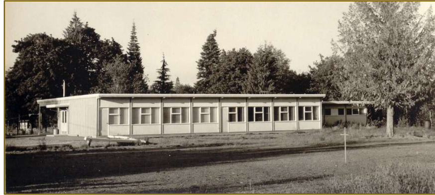
Gibbins Road School, c. 1962
